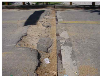
Figura 6. Falla unión soldada en junta de acero. Soldaduras intermitentes Figure 6. Welding failure of steel joint. Non continuous welding
